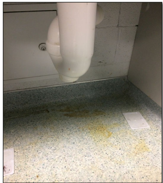
Figure 4: Stained and unsanitary exam room floor
