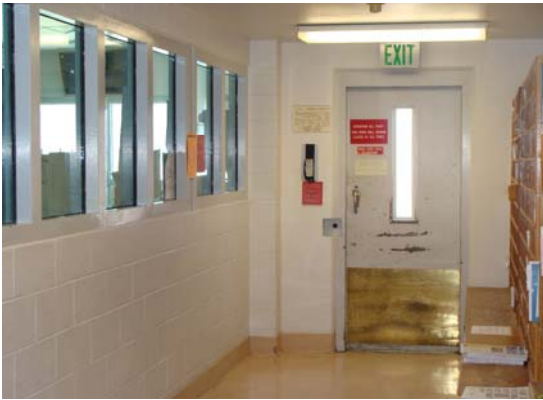
Figure 2 – Secured entry portal into the COC building
