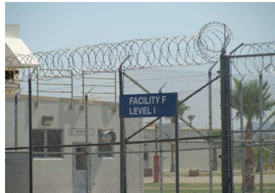
Figure 4 - New fencing installed on CVSP's minimum support yard
